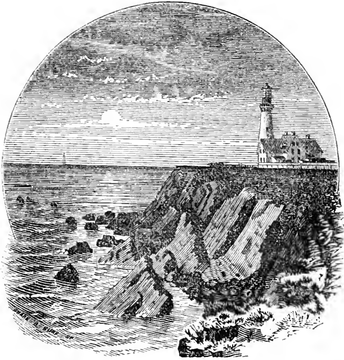
POINT ARENA LIGHT HOUSE.
